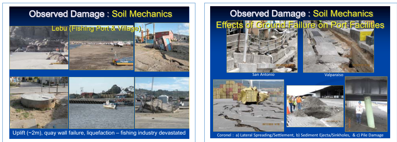
Figure 21 Soil failures in port facilities.
