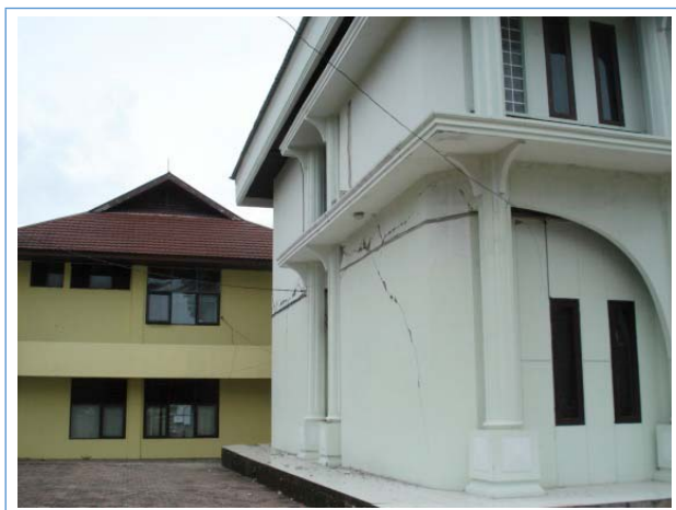
Figure 1 Damage to partition walls
