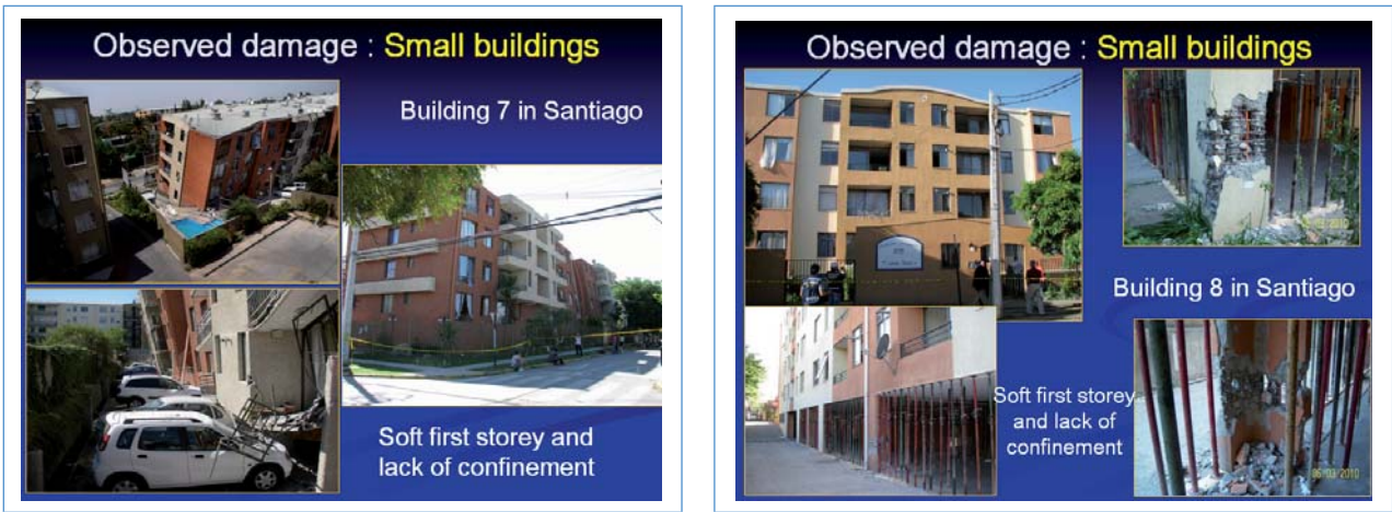
Figure 15 Typical failures due to lack of confinement in compressed wall heads and thin walls
