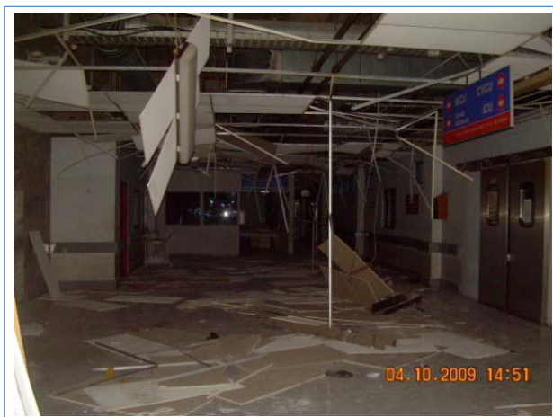
Figure 5 Damage to ceilings
