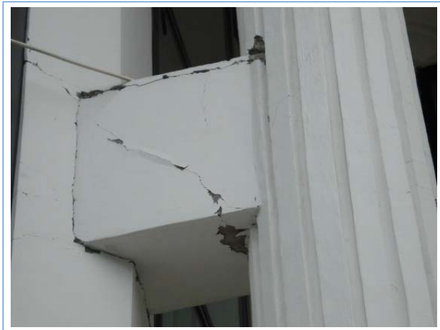
Figure 3 Structural damage to beams and columns
