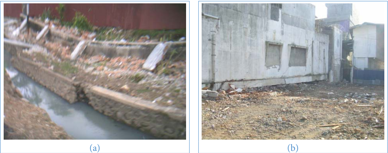
Figure 2 Liquefaction: (a) deformation of the soil layer due to the river wall breaking, Jl. Gereja, and (b) differential settlement of subgrade foundations
