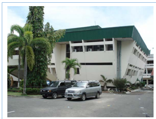
Figure 8 Poor distribution of mass
