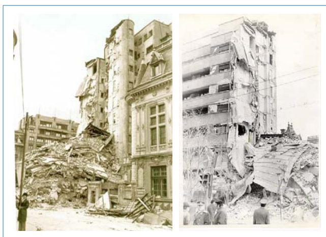
Figure 6 Typical collapse of pre-war tall reinforced-concrete buildings
