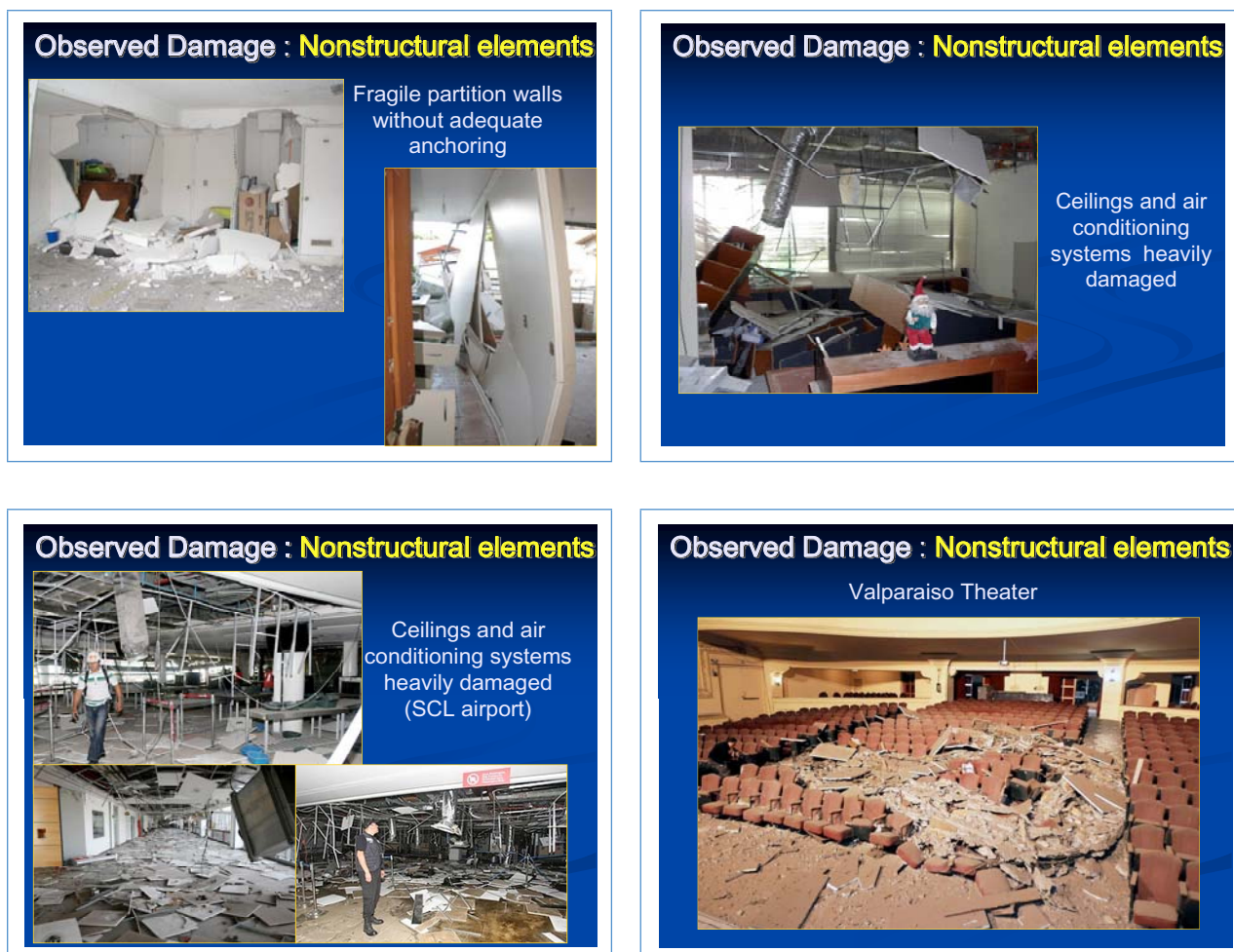
Figure 16 Typical damage to non-structural elements
