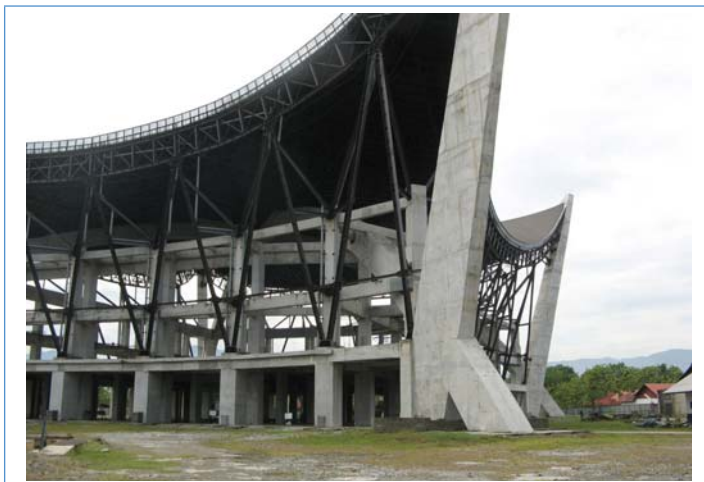
Figure 2 Mosque under construction, surviving intact
