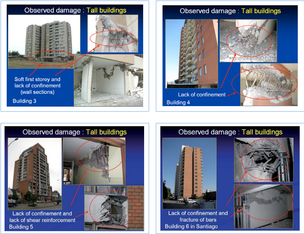
Figure 14 Typical failure due to lack of confinement in compressed wall heads
