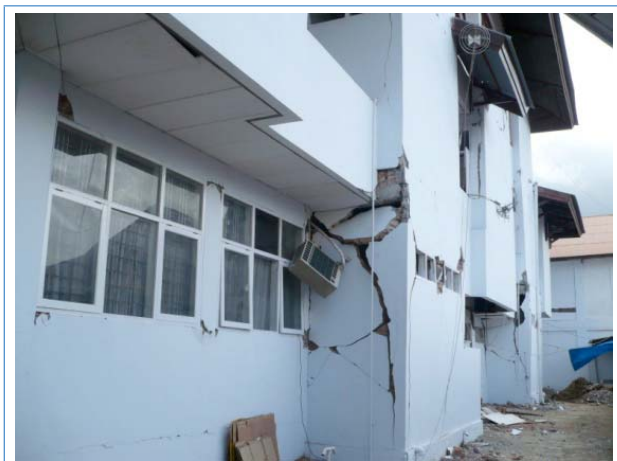
Figure 4 Damage to partition walls
