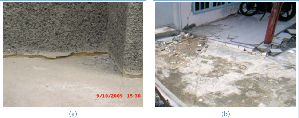
Figure 1 Liquefaction: (a) soil settlement at Jl.Gereja, and (b) sand ejected from the fissure floor in the residential complex at the National University of Padang
