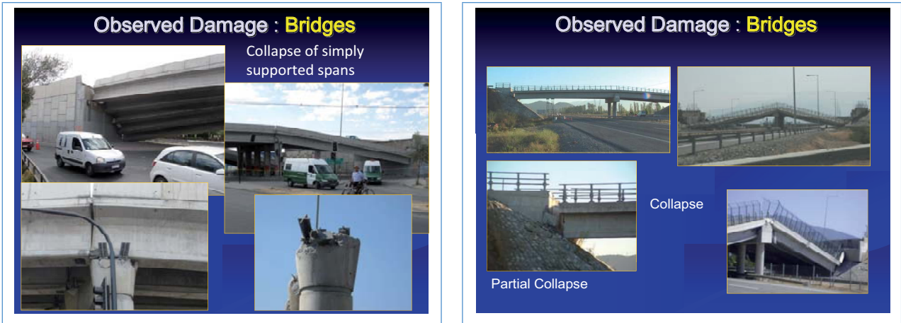
Figure 18 Bridge failure due to weak anchoring and lack of lateral support
