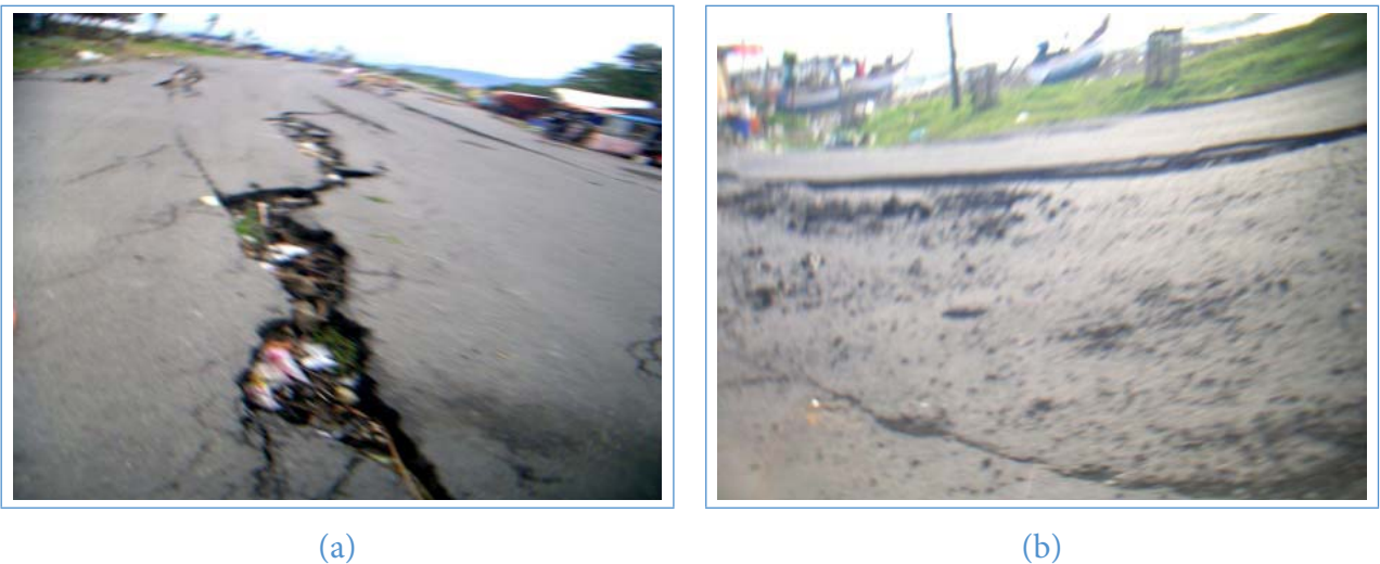
Figure 3 Liquefaction: (a) lateral movement causing a road to crack, Jl. Samudera, and (b) sand from the bottom of a road experiencing landslides, Jl. Samudera
