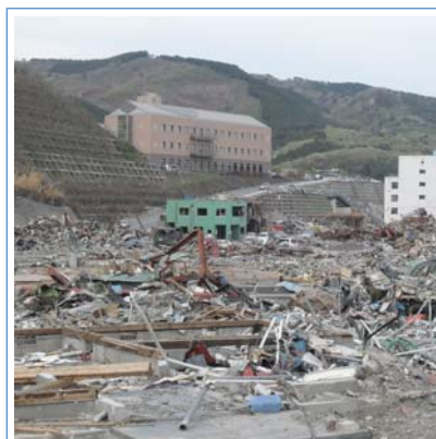
(a) Onagawa Town hospital
