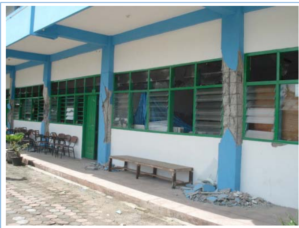
Figure 7 Short column effect
