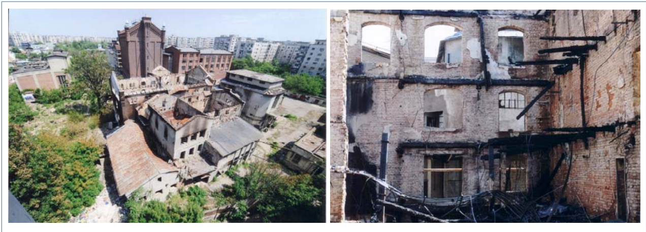
Figure 17. Arson and vandalism precipitated the self-collapse of the Asan Mill, industrial heritage, Bucharest, 1853
