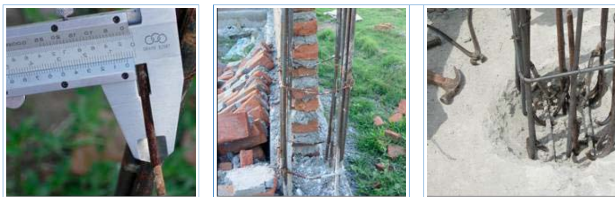
Figure 5 The use of a 4 mm stirrup (left), large spacing of stirrups (centre) and no seismic hook (right)
