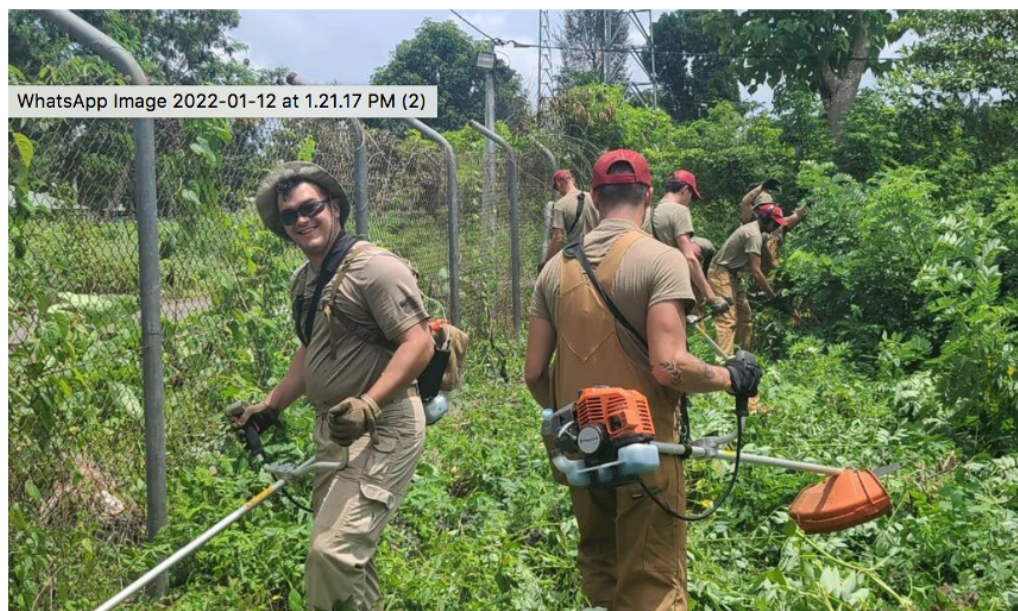
Photo 5: U.S. Air Force Engineers work in partnership with F-FDTL to Rehabilitate Baucau Airfield
