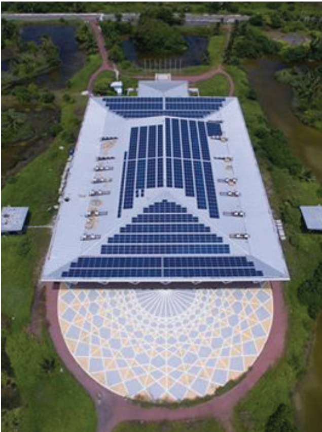
Photo 6: Solar Photovoltaic Installations at Addu City
