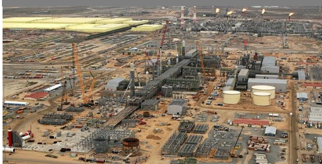
Figure 9: Tengiz: oil production expansion project in Kazakhstan
