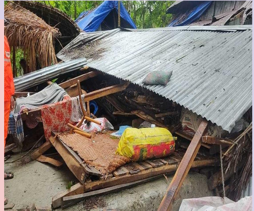
Figure: Damaged House
