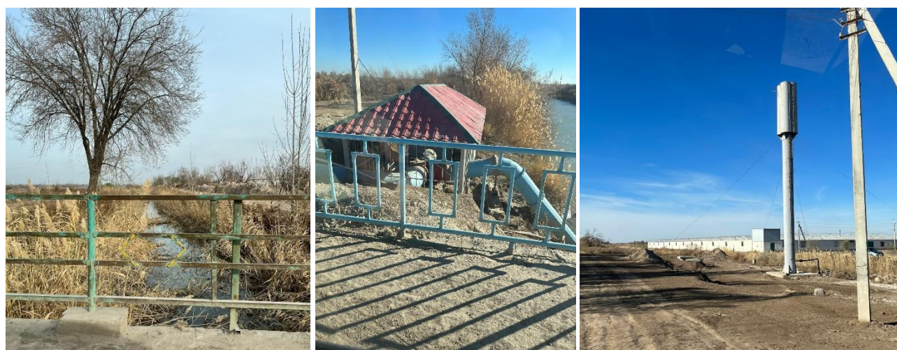
Figure 12: A larger privately managed channel (Yarmas Canal with a capacity of 10m 3 /s; left), a water pump at the farm border providing water for the farm from the public channel (middle), a farm-owned water tower used as small reservoir (right)
