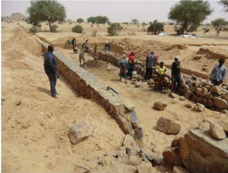
Image 1: Installation of the water-spreading weirs
