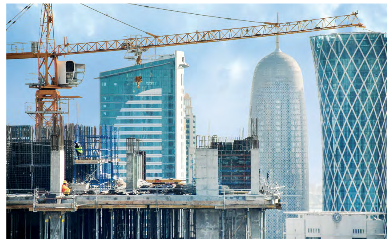
Construction of skyscrapers, Doha
