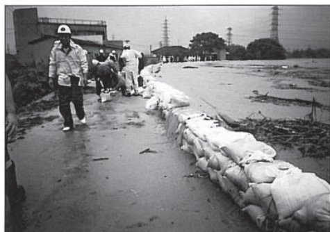
"Sandbag piling technique (Tsumidono ko)" (Torrential Rain in Niigata and Fukushima in 2004) The Ikarashi River in Niigata Prefecture
