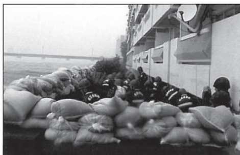
"Sandbag piling technique (Tsumidono ko)" (Typhoon No. 14 in 2005) The Ooyodo River in Miyazaki Prefecture
