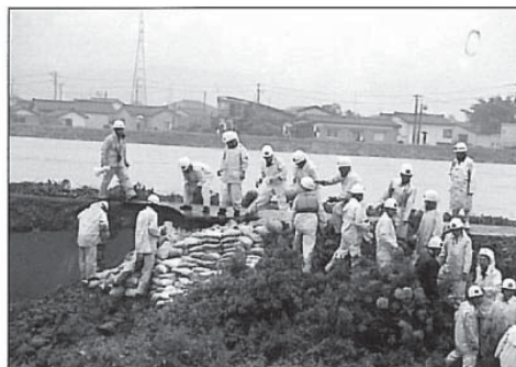
"Sandbag piling technique (Tsumidono ko)" (Torrential Rain in Niigata and Fukushima in 2004) The Ikarashi River in Niigata Prefecture
