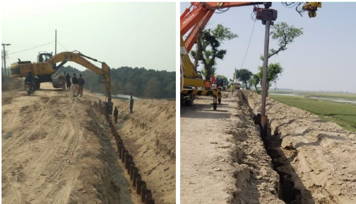
Picture 4: Steel sheet piling to enhance resilience of Nawabpur Flood Bund and LMB Taunsa, Punjab
