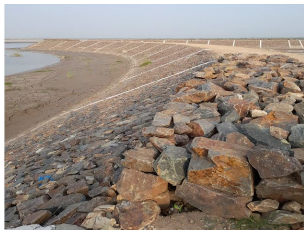
Picture 3: Spur with earthwork, stone apron, stone pitching, and shingle on top of spur in Kalowal Gujrat, Punjab
